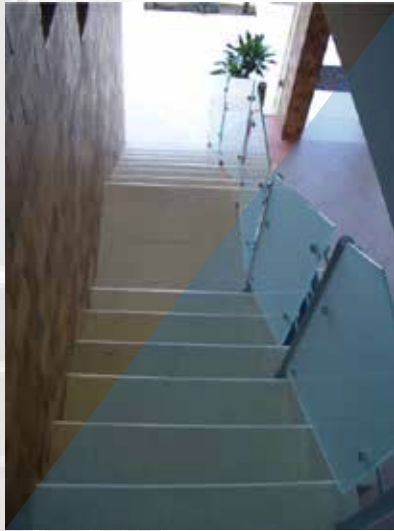
Balustrade: 15 mm Tempered Glass + Stainless Steel Handrail.
