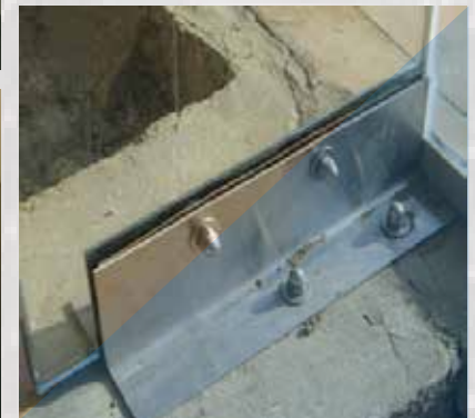
12 mm Tempered Float Glass
