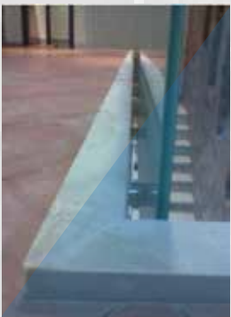
Balustrade: 15 mm Tempered Glass + Stainless Steel Handrail.
