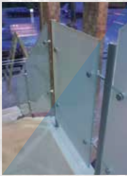
Balustrade: 15 mm Tempered Glass + Stainless Steel Handrail.
