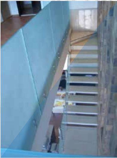
Balustrade: 15 mm Tempered Glass + Stainless Steel Handrail.
