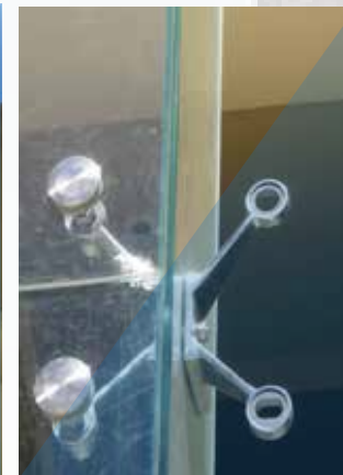
12 mm Tempered Float Glass
